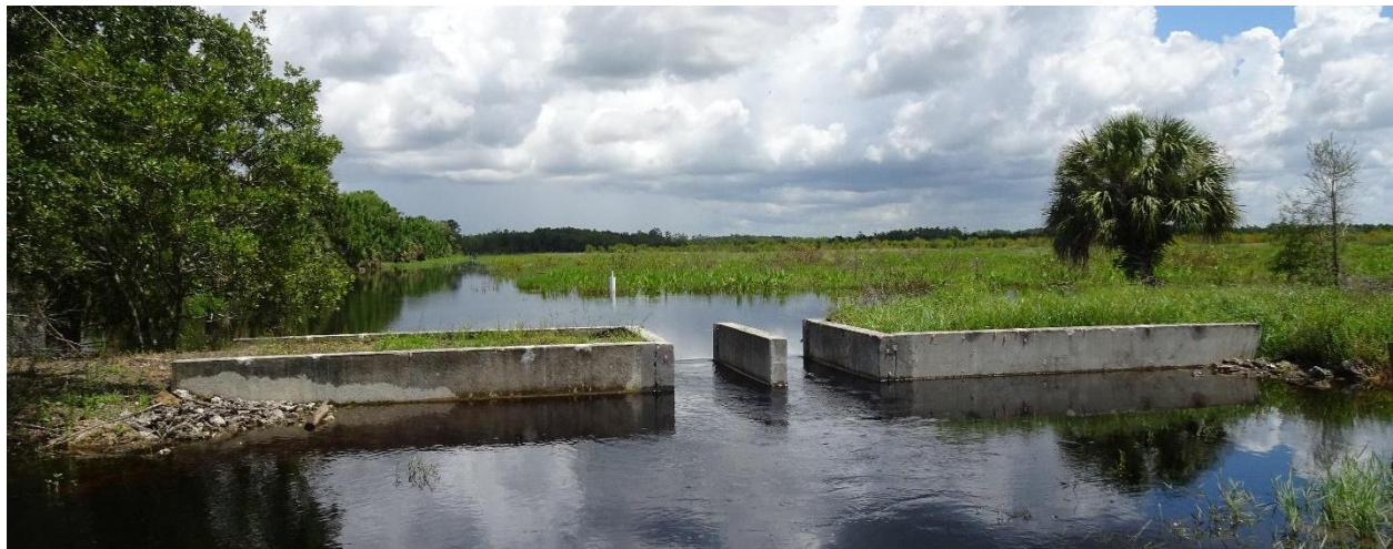
Figure 19. Corkscrew Mitigation Bank Outfall, August 8, 2019
