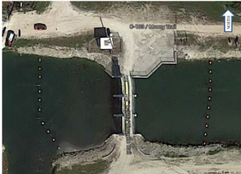
Figure 1 – Aerial image of the S20F Structure site
