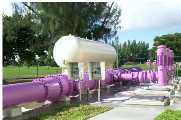
Figure 6-3: Reclaimed Water System
