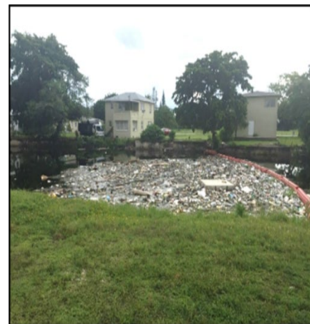
Trash build-up in the C-7 Canal.
