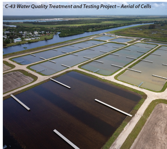
C-43 Water Quality Treatment and Testing Project – Aerial of Cells
