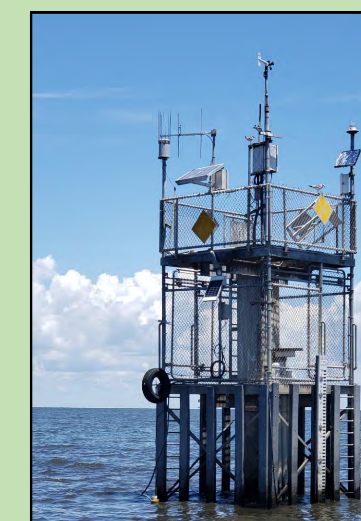
Lake Okeechobee instrumentation platform and telemetry tower.
