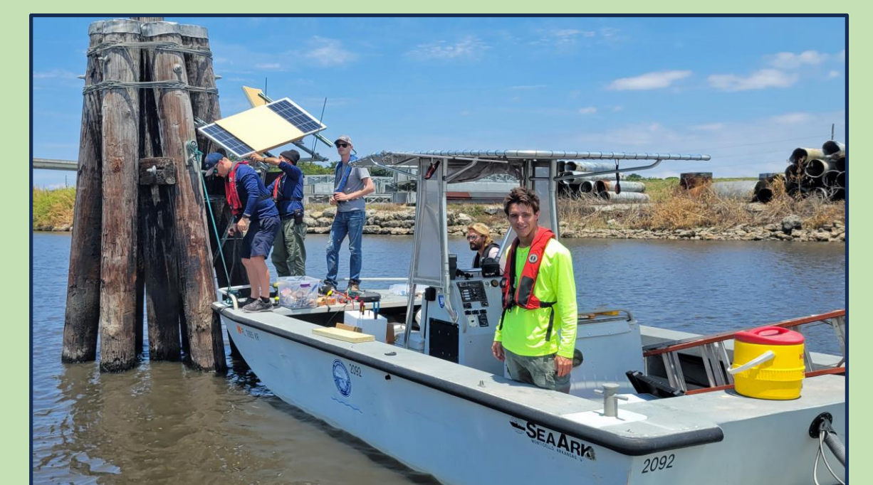
S-308C channel marker on Lake Okeechobee. Installing solar panels to power the deployed continuous monitoring equipment.
