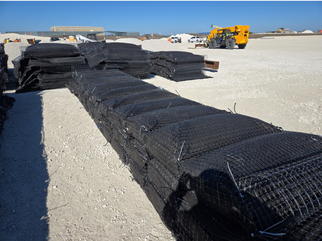
Photo 7 B&Z installing marine mattresses, low sill weir at appx STA 0+53, L-29 canal.
