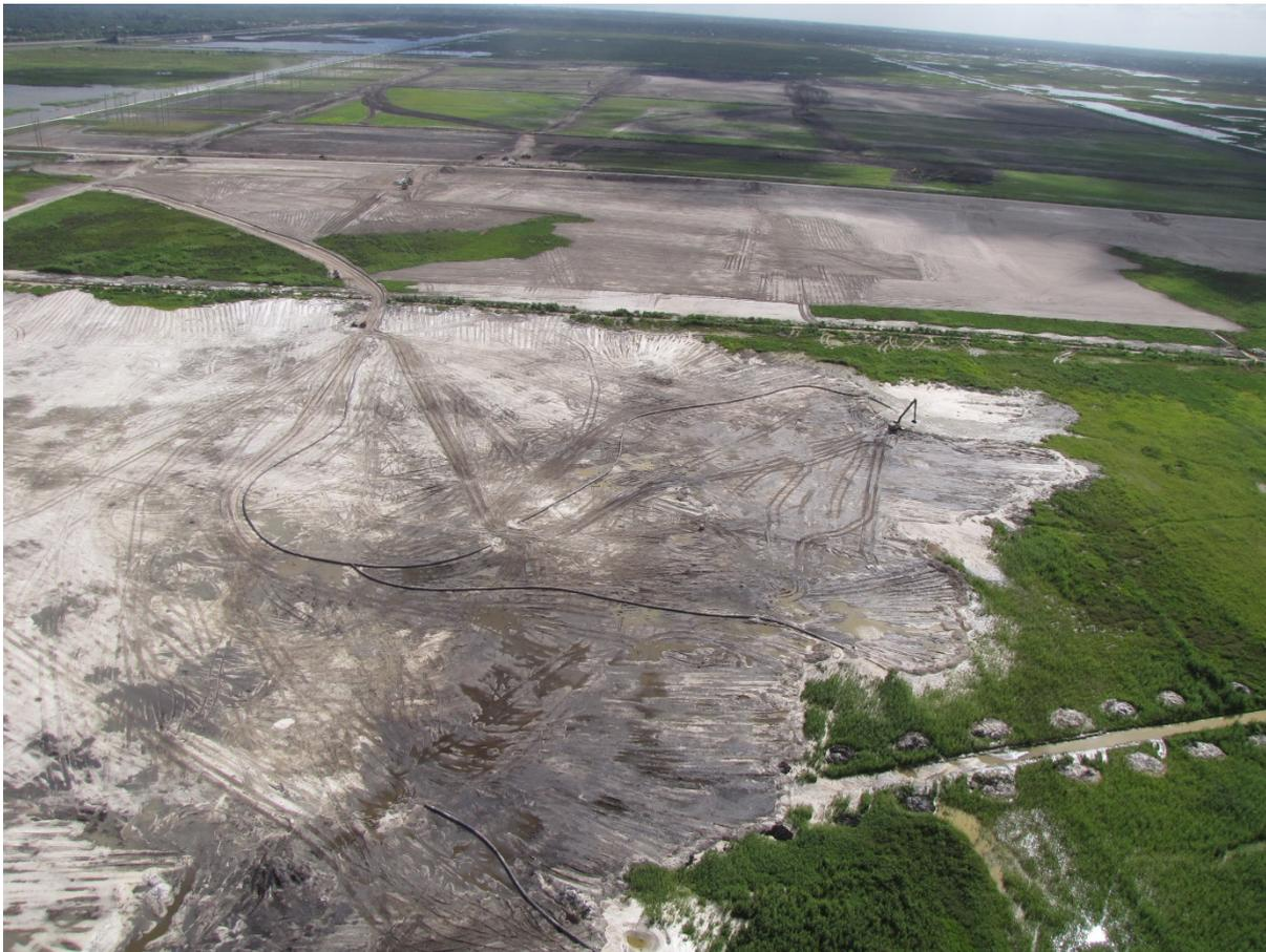
Earthwork for STA-1E Improvements. Photo illustrates the re-distribution of fill dredged from WDC in Cell 7. The regrade of Cell 5 can be seen in the background
