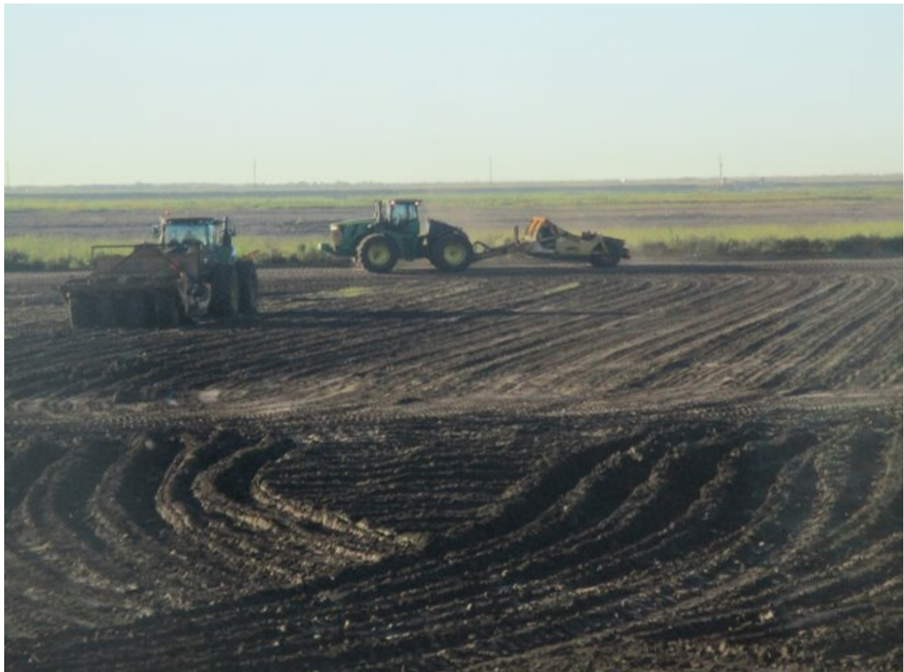
Earthwork for STA-1E Improvements. Photo illustrates re-grading in Cell 5.
