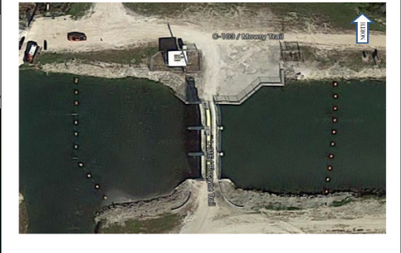
Figure 1 – Aerial Image of the S20F Structure site
