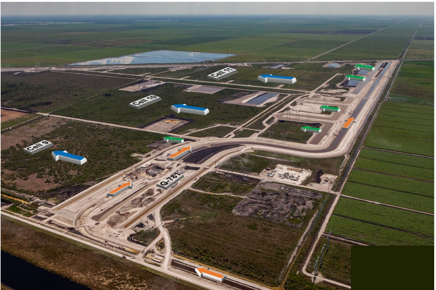
Southwestern aerial view of STA -1W Expansion #2 under construction
