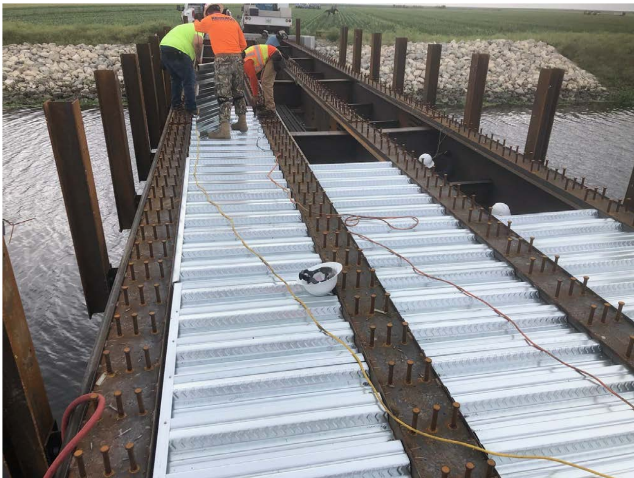
G-341 Conveyance Improvements: Installation of steel superstructure at the Jett Farm Bridge
