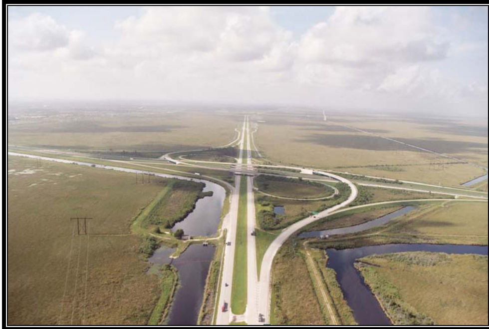
Photograph 1 – Aerial view of the northern section of the project area. View toward the south.
