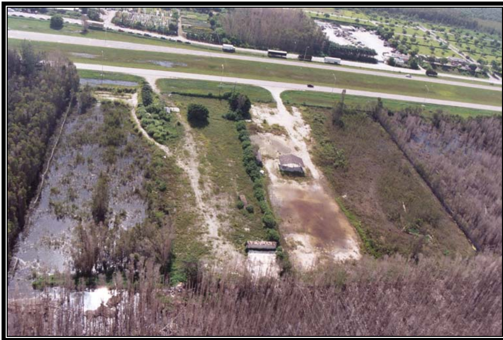
Photograph 12 – Aerial view of Tract 9312-003 (Carpomex of America/Cruz Property) and Tract 9312-025 (Montenegro Equipment Service/Delta Holdings Property). View toward the east.
