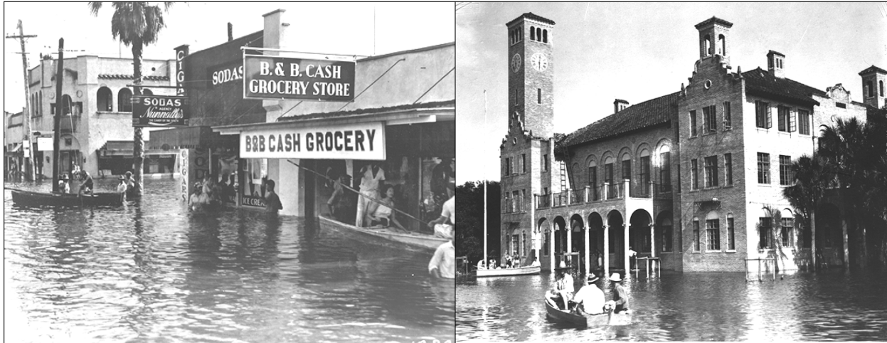
Figure 3. 1948 Flood event in the city of Kissimmee.
