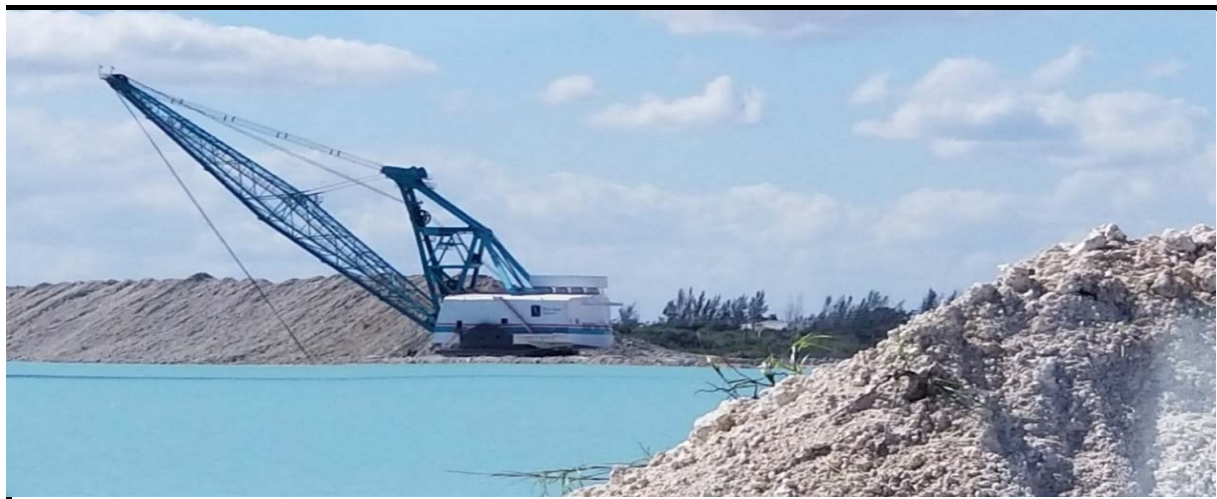
Excavated above ground limerock pile
