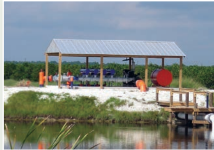
Surface Water or Tailwater Irrigation Pumps and Filters
