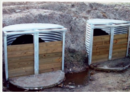
Riser Culverts and Water-Control Structures
