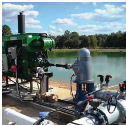
Surface Water Wet Well and Engine
