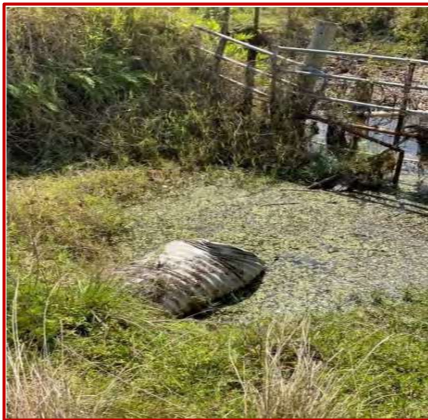
Damaged culvert near cattle pens
