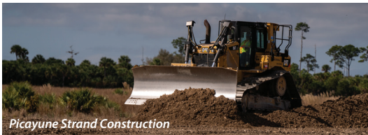
Picayune Strand Construction
