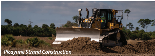
Picayune Strand Construction
