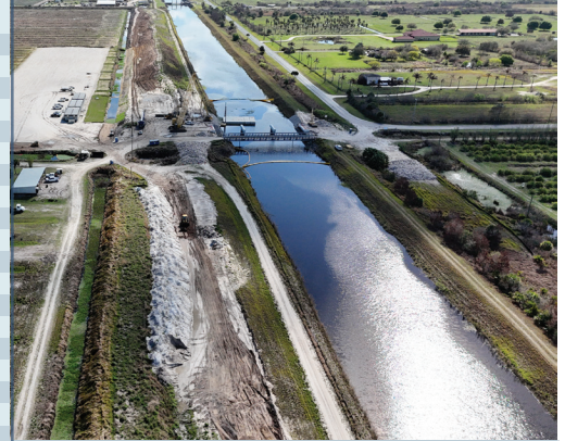
C-25 Clearing and Construction
