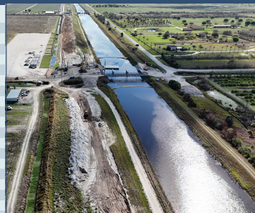
C-25 Clearing and Construction
