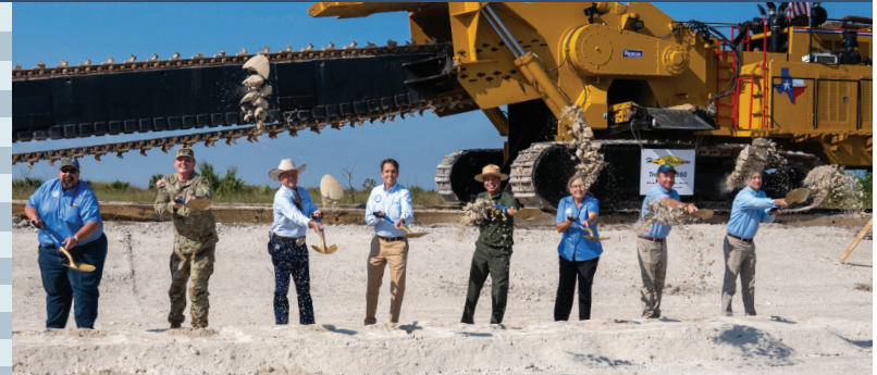
CEPP New Water Seepage Containment Wall Groundbreaking Ceremony
