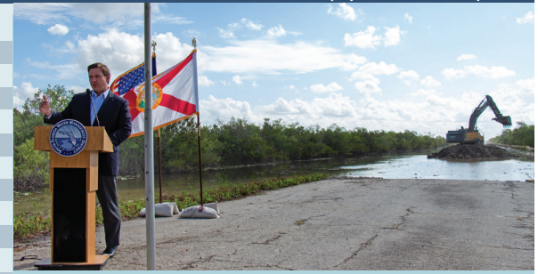
Gov. DeSantis at the Old Tamiami Trail Roadbed Removal Groundbreaking
