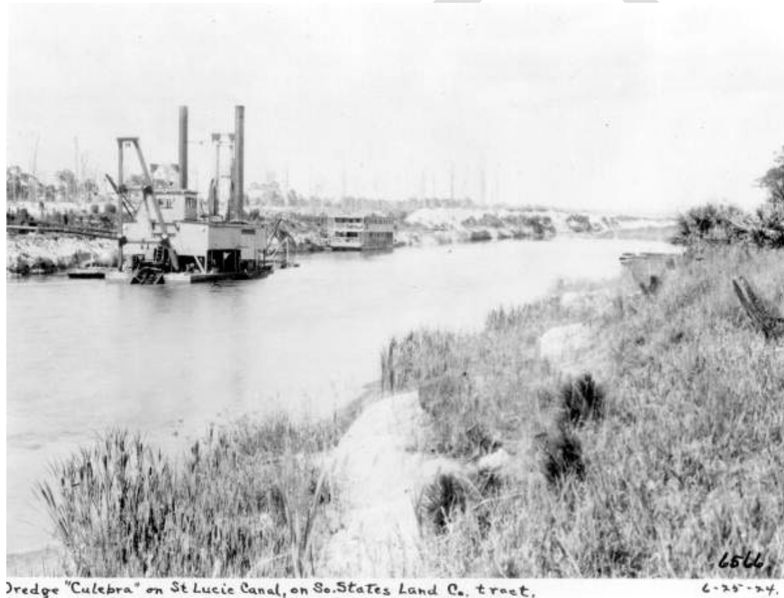
Figure 6. 1924 Photograph of the St Lucie Canal Dredging.
