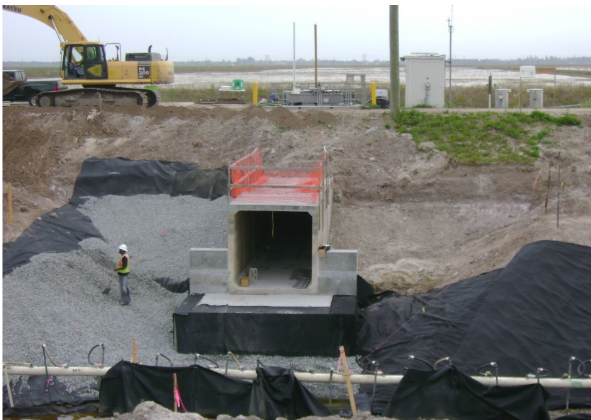
Figure 5A-6. STA-1E Culvert Repairs.
