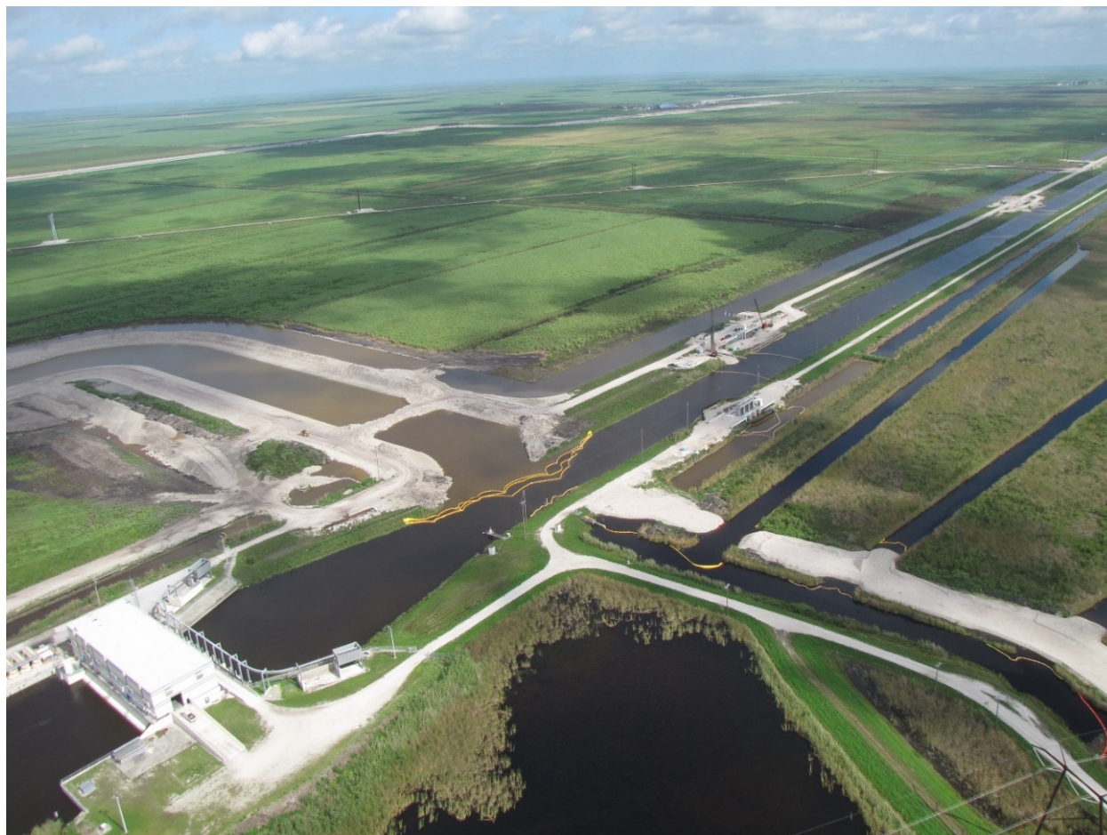
Figure 5A-3. STA-1W Outflow Pump Station G-310 with structures and canals being constructed as part of STA-1W Expansion #1, looking northwest (photo by SFWMD, May 2018).
