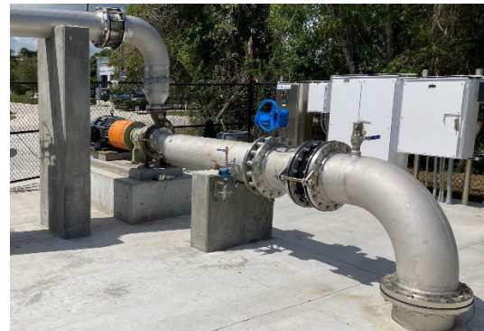
Newly Constructed Floridan Aquifer System Well
