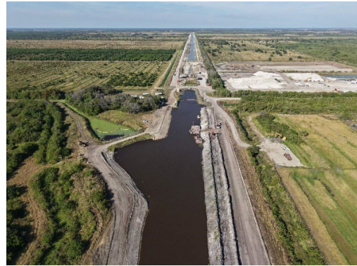
C-23/C-24 South Reservoir – Construction in Progress as of December 2025
