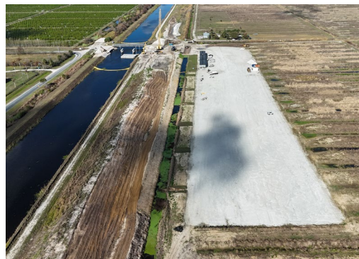
C-25 Reservoir and STA – Construction in Progress as of February 2026
