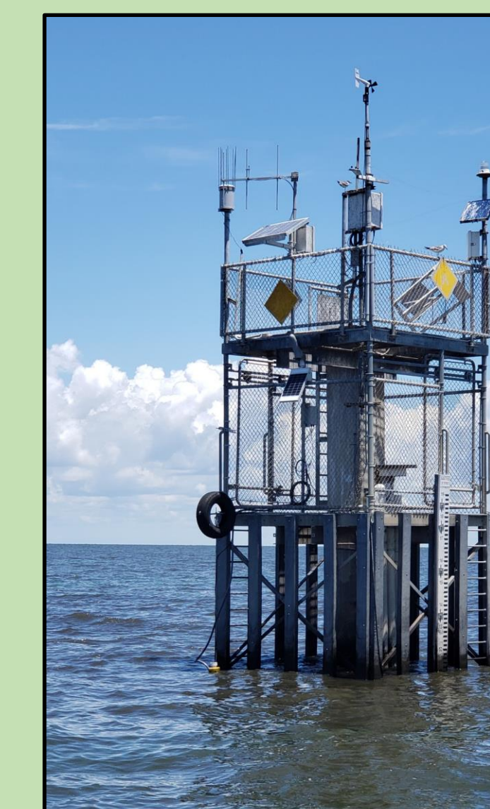
Lake Okeechobee instrumentation platform and telemetry tower
