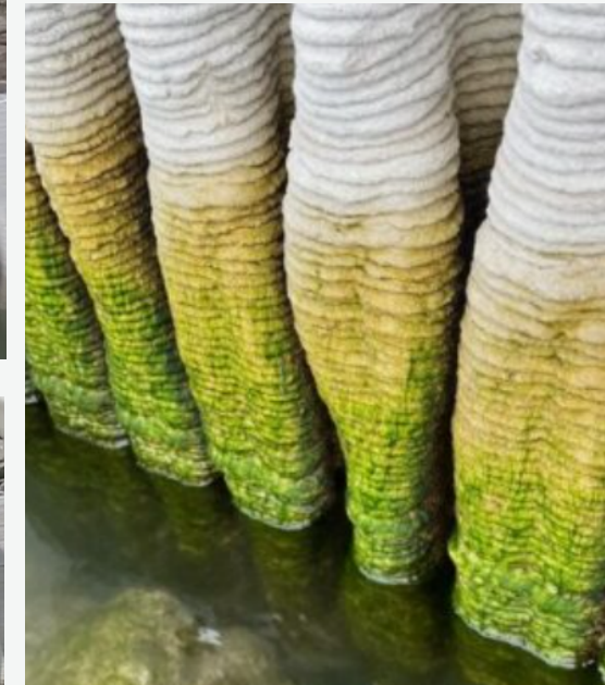
Sample Marine Growth on Seawall
