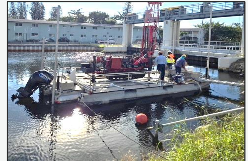
Geotechnical Investigation at Existing S-27 Spillway
