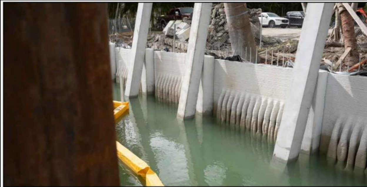
KIND DESIGNS PRE-CAST CONCRETE BATTER PILE SEAWALL
