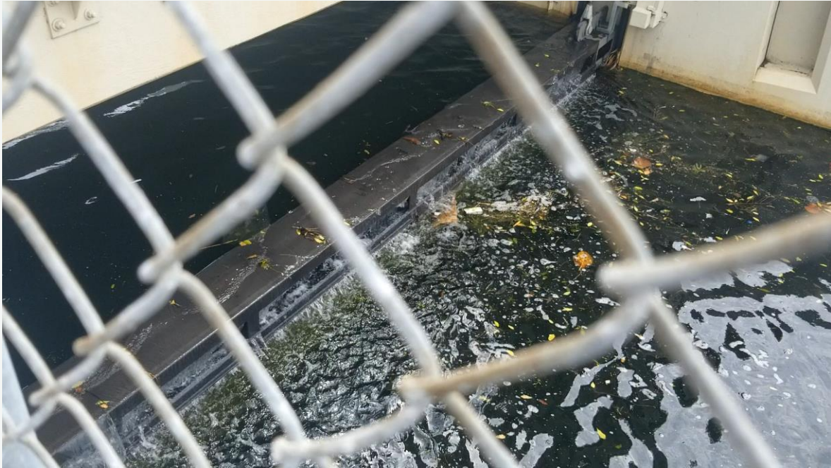
Coastal Structure Gate Overtop (Saltwater moving inland, bypassing the top of the gate of the salinity coastal structure) High Tide Season 2019
