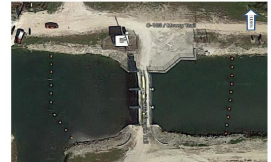
Figure 1 – Aerial Image of the S20F Structure site
