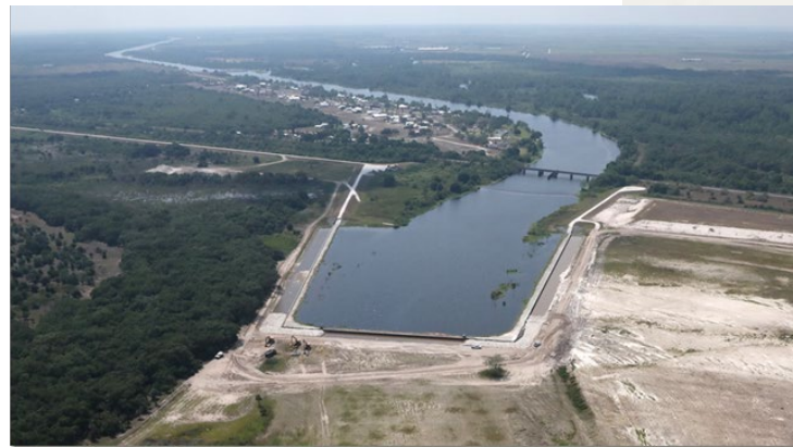
CNT 12A – S69 Weir ongoing repair work
