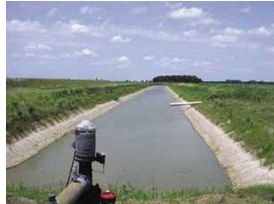
Tailwater recovery system
