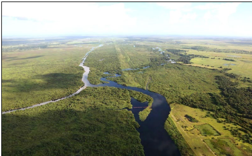
Kissimmee River Restoration Project (KRRP): Looking north from the south end of the Phase I restoration area.
