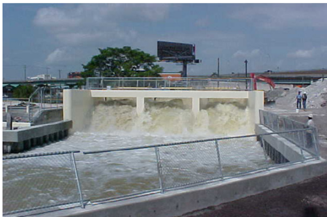
Forward pump assist gravity structure to discharge stormwater at S-26, Miami-Dade County.
