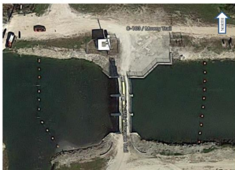
Figure 1 – Aerial image of the S20F Structure site
