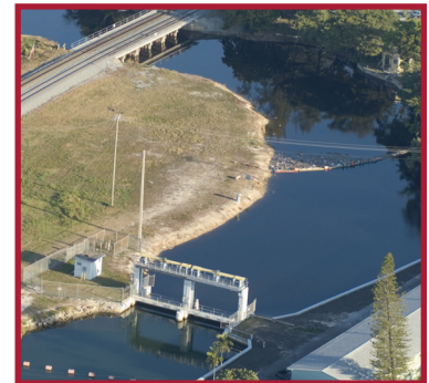
S-27 Structure Gate.
