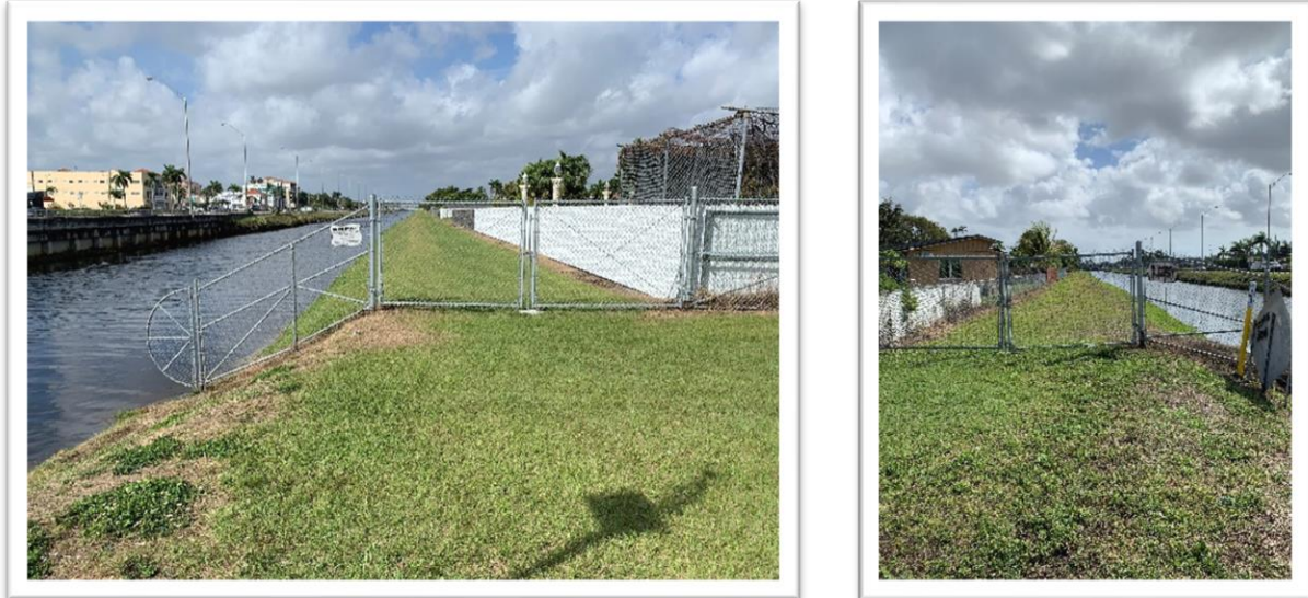
Figure 3-3 – Site Conditions at the C4 Flood Wall (C4.CORAL)
