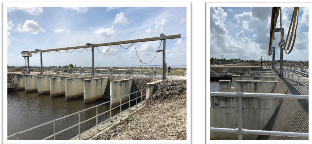
Figure 3-10 – Site Conditions at the G-422 Structure
