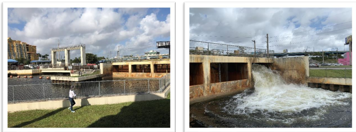
Figure 3-2 – Site Conditions at the S-26 Structure
