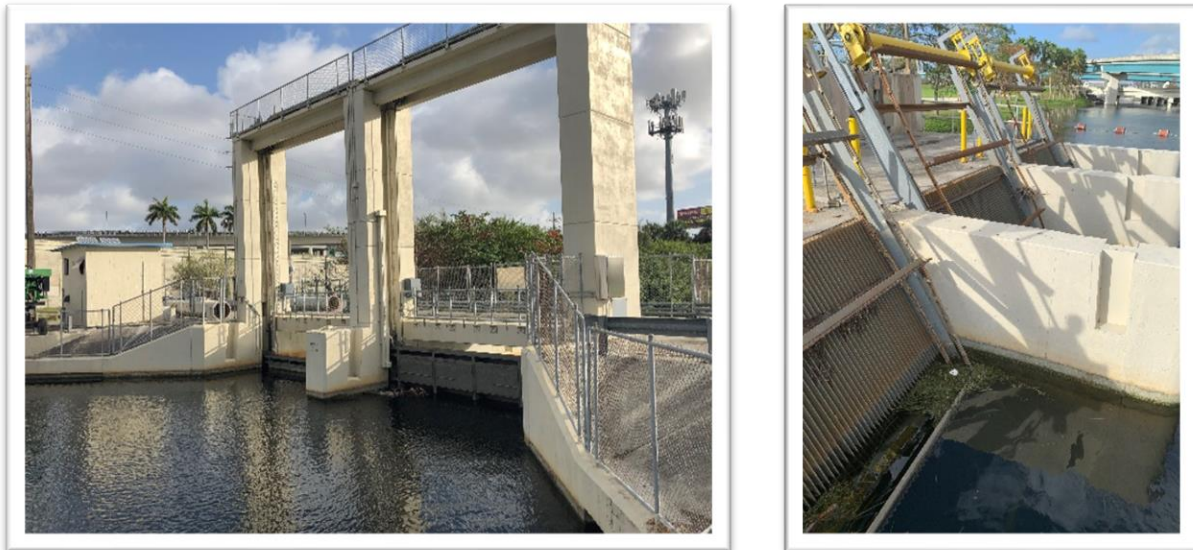
Figure 3-1 – Site Conditions at the S-25B Structure
