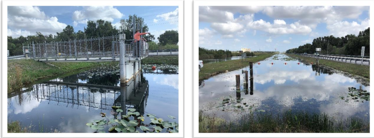
Figure 3-11 – Site Conditions at the S-336 Structure
