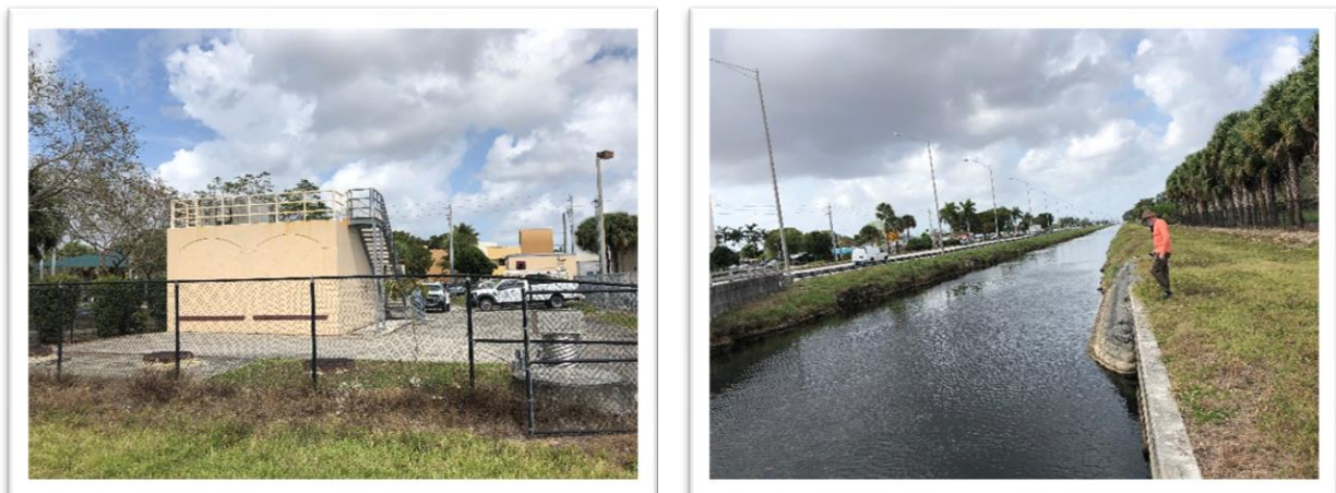
Figure 3-4 – Site Conditions at the Belen Pumps
