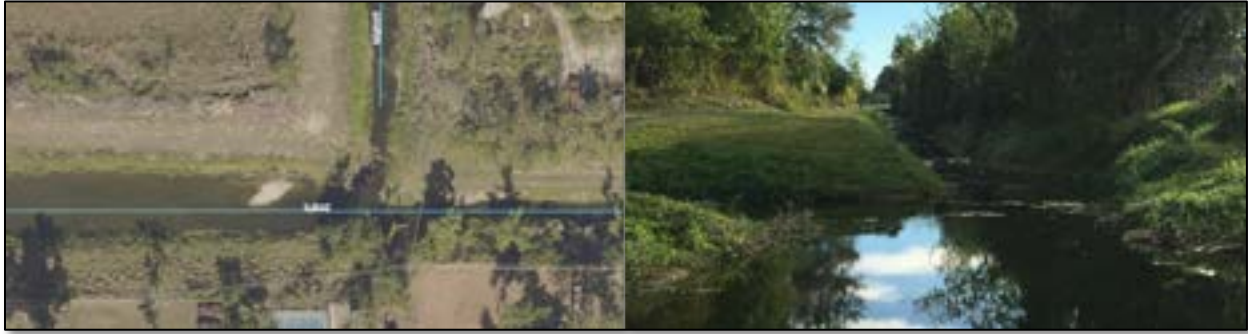
Figure 8. Aerial and Ground Views of the Constricted Area in L Canal between L-3 and Tamiami Trail
