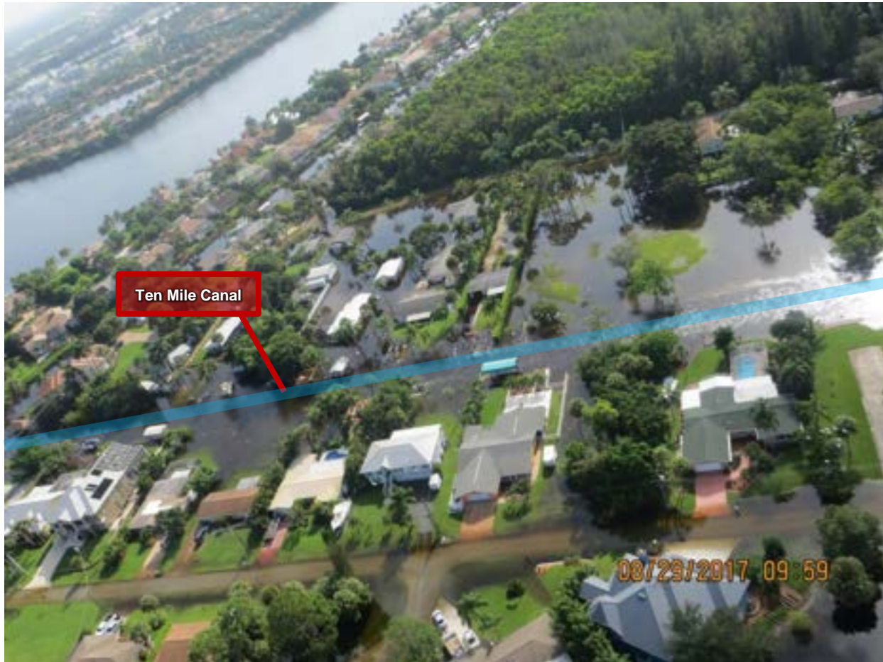
Figure 10 - Example of the limited Ten Mile Canal conveyance and canal bank flood-stage exceedance.
