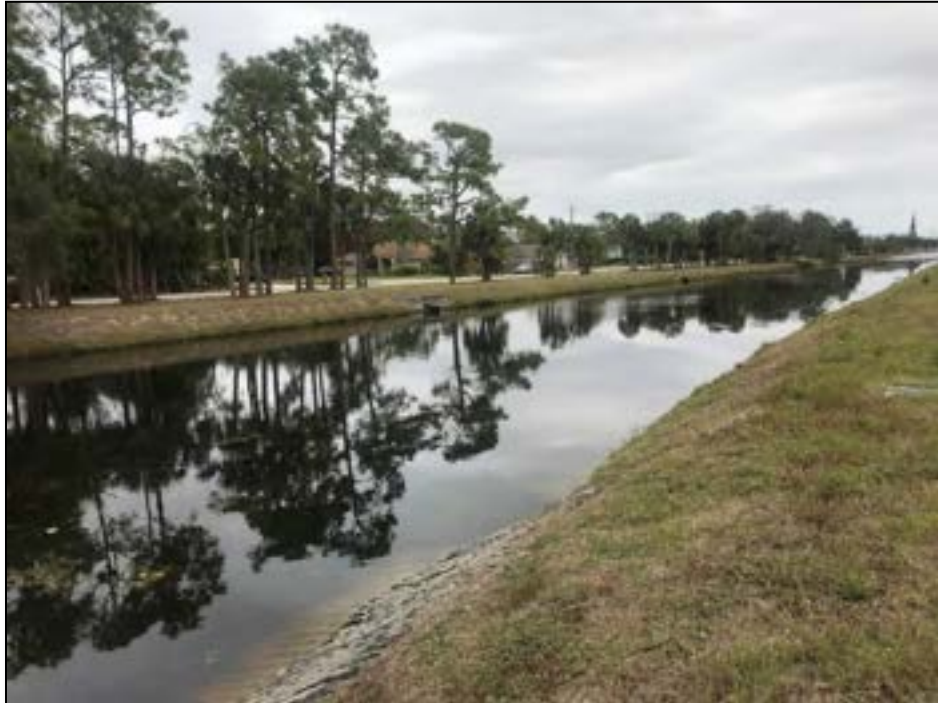
Figure 3 – Example of a high flow drainageway channel conveyance
