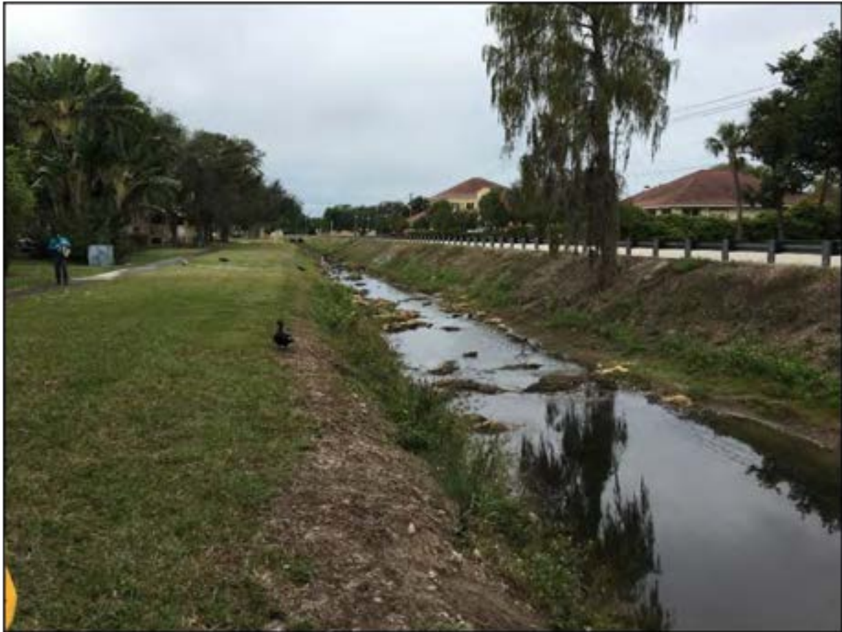
Figure 12 - Photo of BDC Canal East of Summerlin Road
