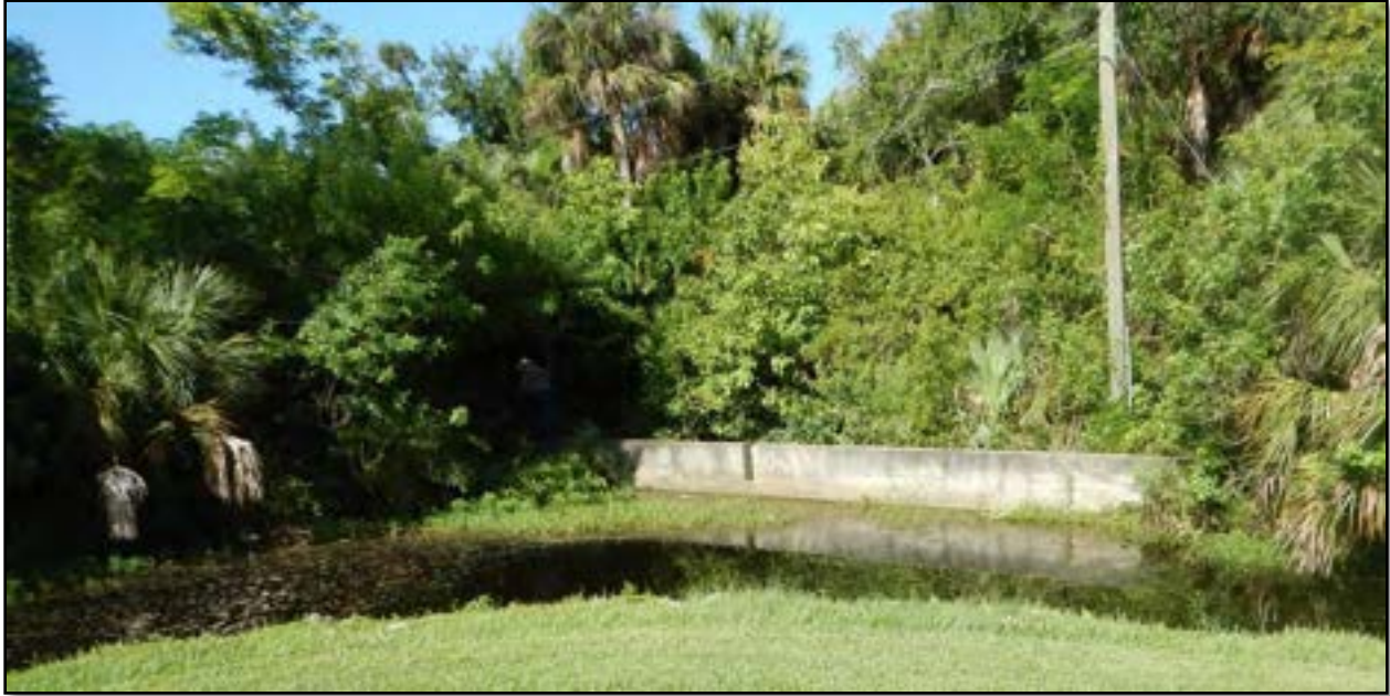
Figure 11 - Existing outfall weir for the Jamaica Bay community.
