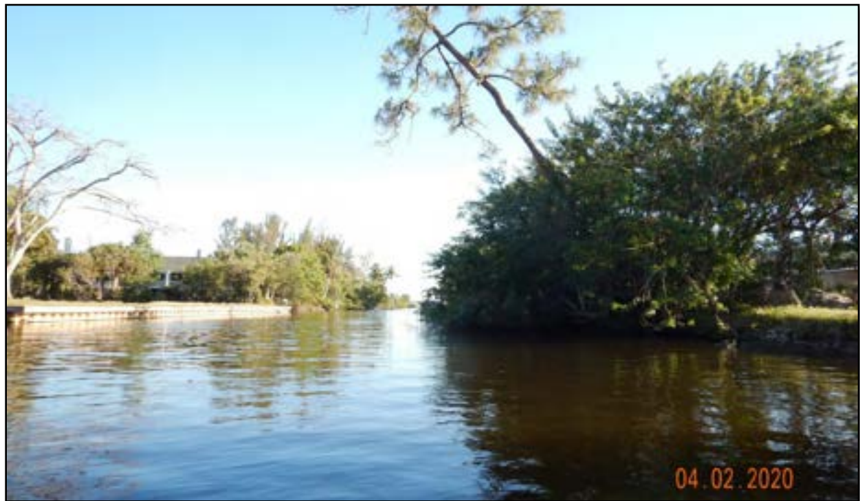
Figure 2 - Example of vegetation obstructions within the channel at STA 127+00, looking south.
