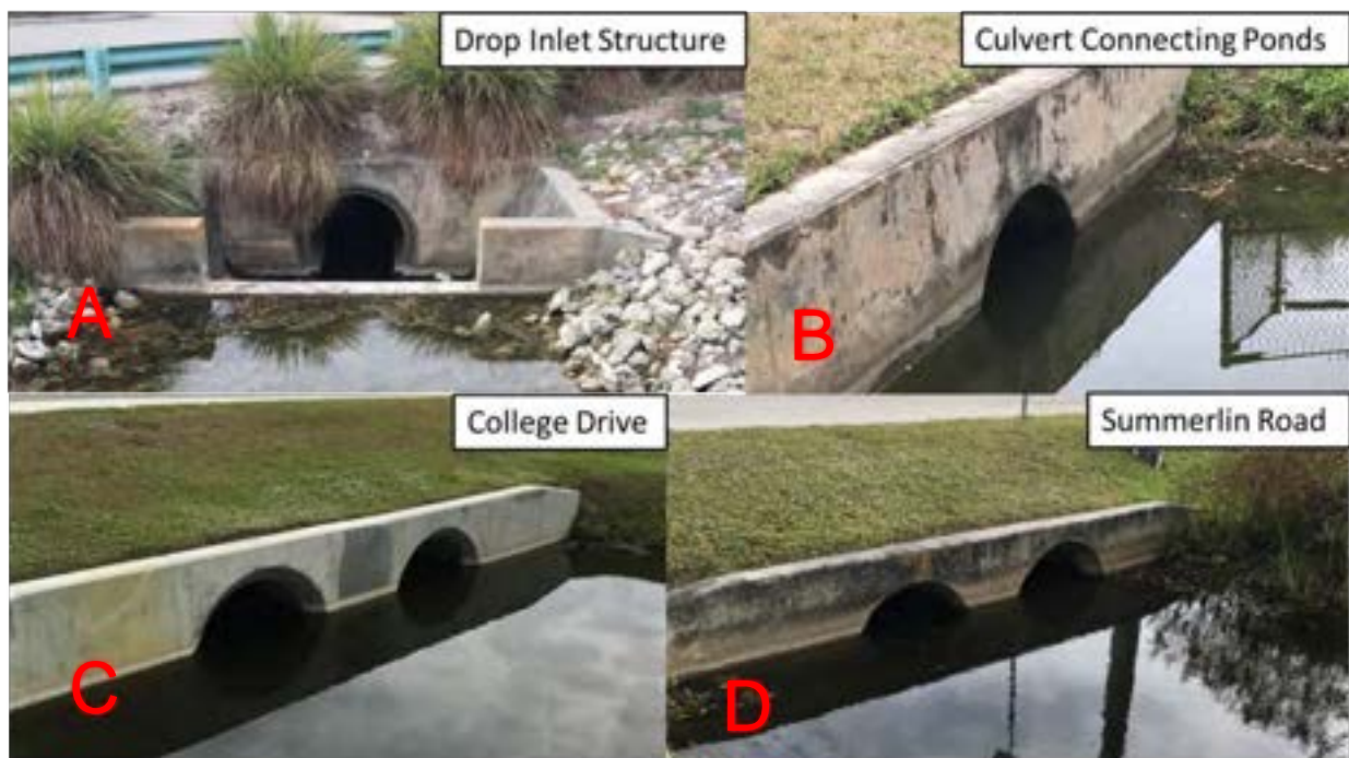
Figure 17 – Photos of Weir Structure and Culverts within FSWSCC Project Area
