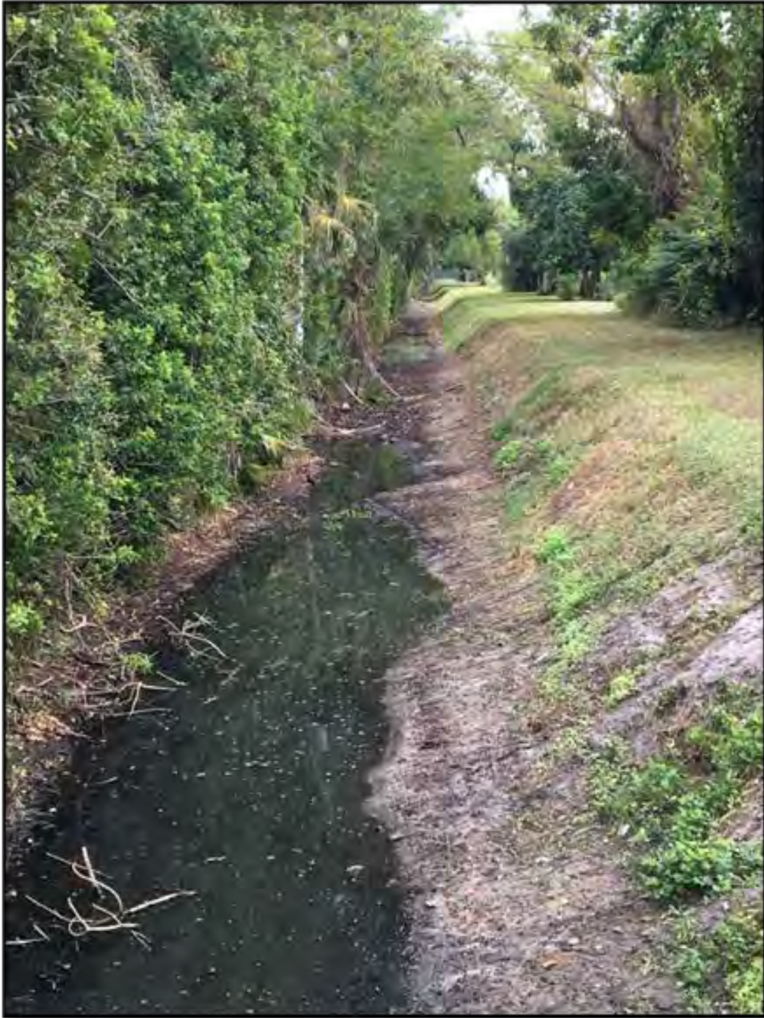
Figure 13 – Photo of BDC Canal East of Tamiami Trail (US 41)
