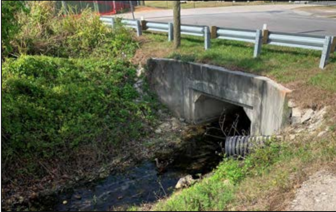
Figure 6 - Existing 7'x4' box culvert crossing of Canal L under 4th Street.
