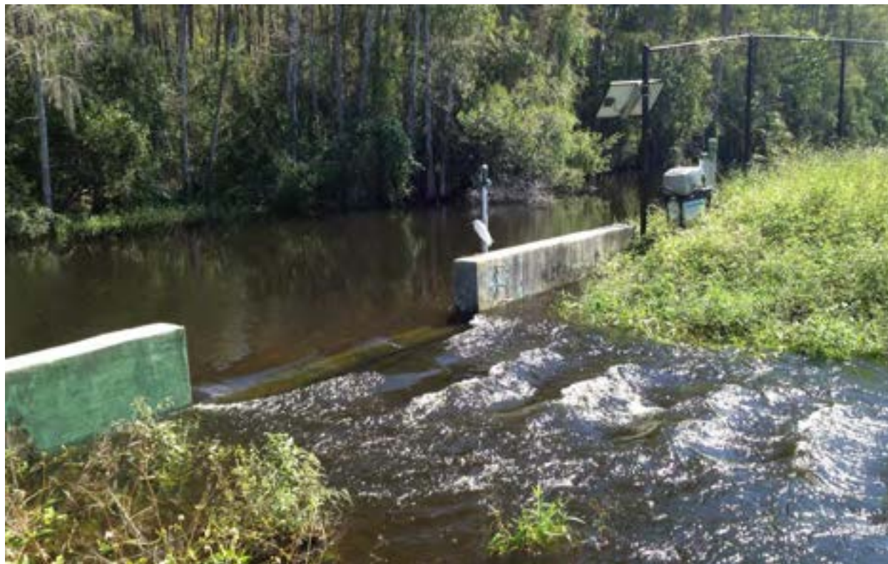
Figure 7 – Example Side-Bank Overflow Spillway Perpendicular to a Canal.
