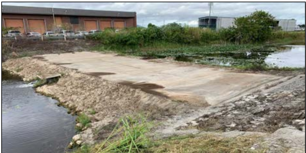
Figure 6 – Existing Weir in Ten Mile Canal West of Page Field Airport.
