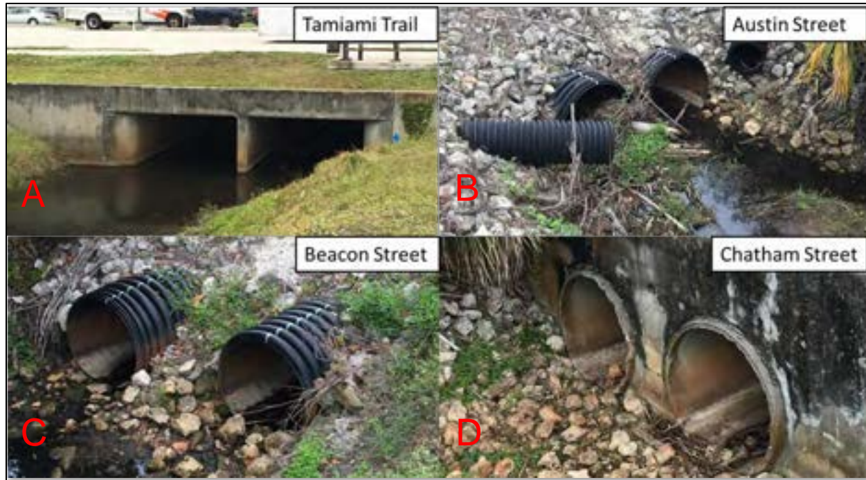
Figure 15.– Photos of Tamiami Trail Box Culverts and Upstream Culverts
