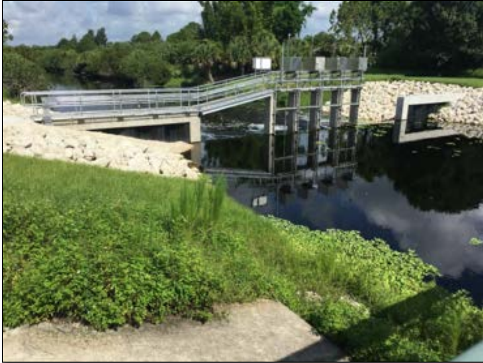
Figure 2 – Example of a water control structure with remote operable gates
