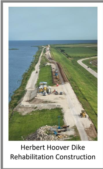
The USACE is rehabilitating the Herbert Hoover Dike, a 143-mile series of levees and structures surrounding Lake Okeechobee, to address structural integrity concerns. The Herbert Hoover Dike was authorized in 1930 and constructed by hydraulic dredge and fill methods. In 2006, the USACE assigned the Herbert Hoover Dike a Safety Action Classification (DSAC Level 1), representing the highest risk of failure and requiring remedial action.
