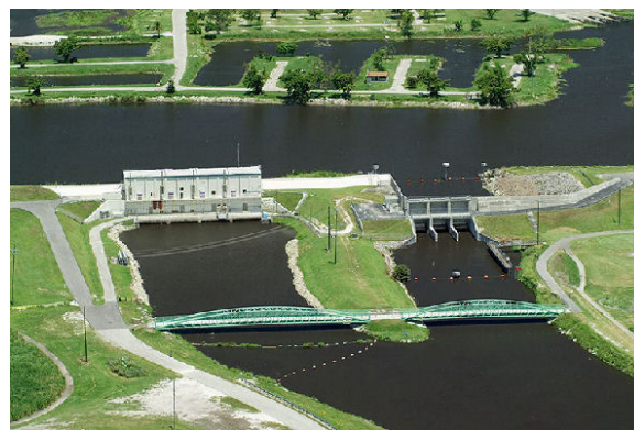
Lake Okeechobee Water Control Structures
