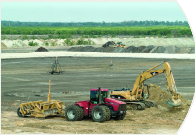
Constructing the C-43 Basin Storage Reservoir.
