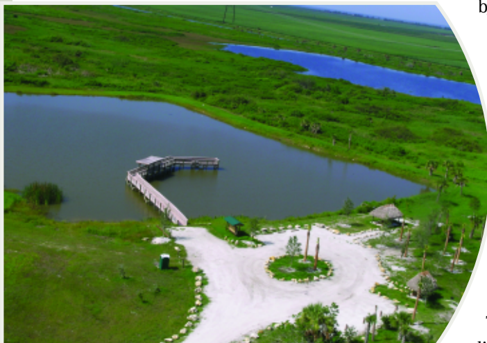
DuPuis Fishing Pier – recently constructed parking and picnic areas.
