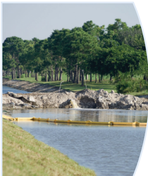
Acme Basin B Discharge Canal along Flying Cow Road in Wellington, Florida
