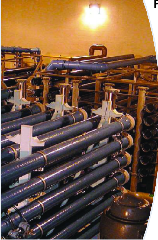
Typical Reverse Osmosis (R.O.) Treatment System
