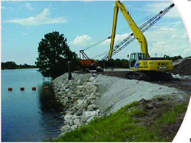
Bank hardening work at District structure S-65E.
