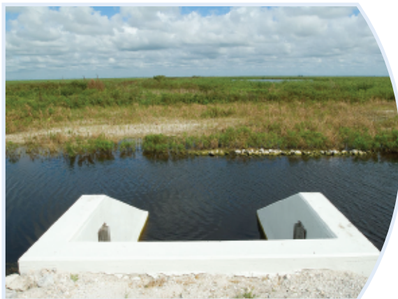
Culverts between cells at STA-1W
