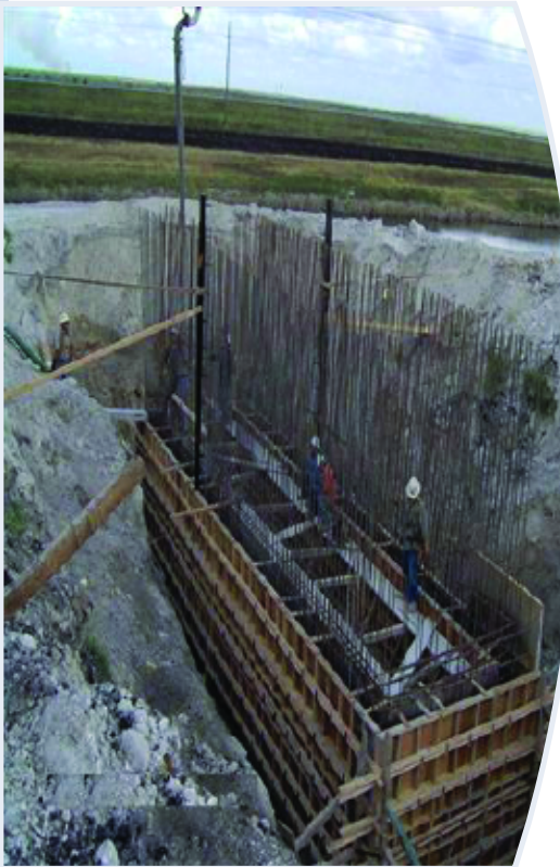
Structure construction for a stormwater treatment area (STA) expansion project.
