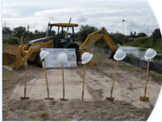
C-44 Reservoir Groundbreaking
