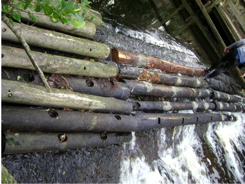
Log installation on the top of Lainhart Dam
