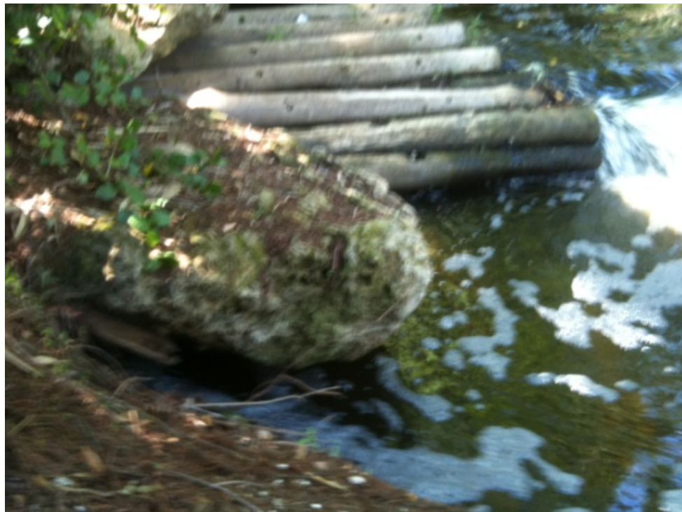
Lainhart Dam - East bank looking southwest, flow under the rock appears to bypass main structure
