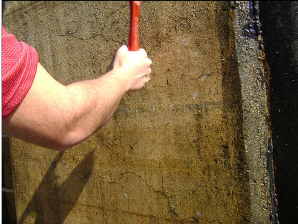
Figure 14. Photograph of the cracked shotcrete surface at S65A. Crack width ranges from hairline to 1/8-inch wide. After South Florida Water Management District, Memorandum on S-65 and S-65A Concrete Repair Cracks, February 14, 2012.
