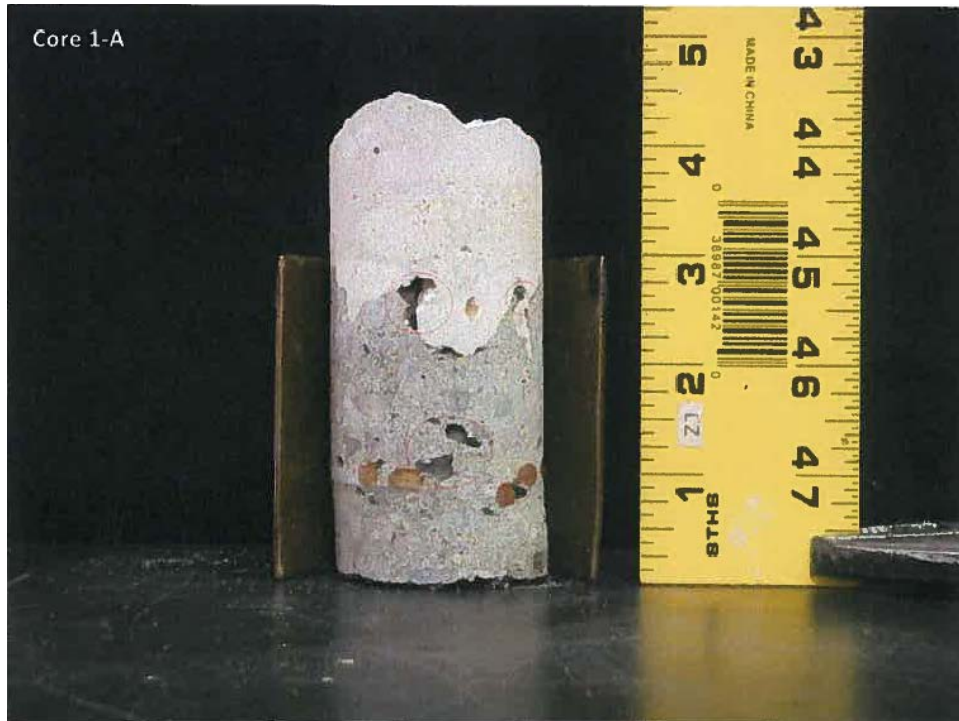
Figure 12. Photograph of a shotcrete core from S-59 Spillway Structure showing 1/16" to 1/2" voids. Some voids occur at the concrete substrate and shotcrete interface. 40
