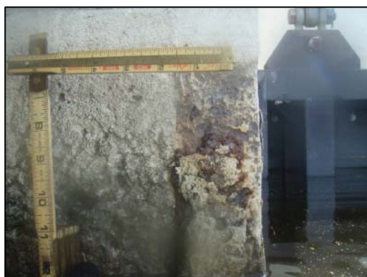
Figure 11. Steel Corrosion
