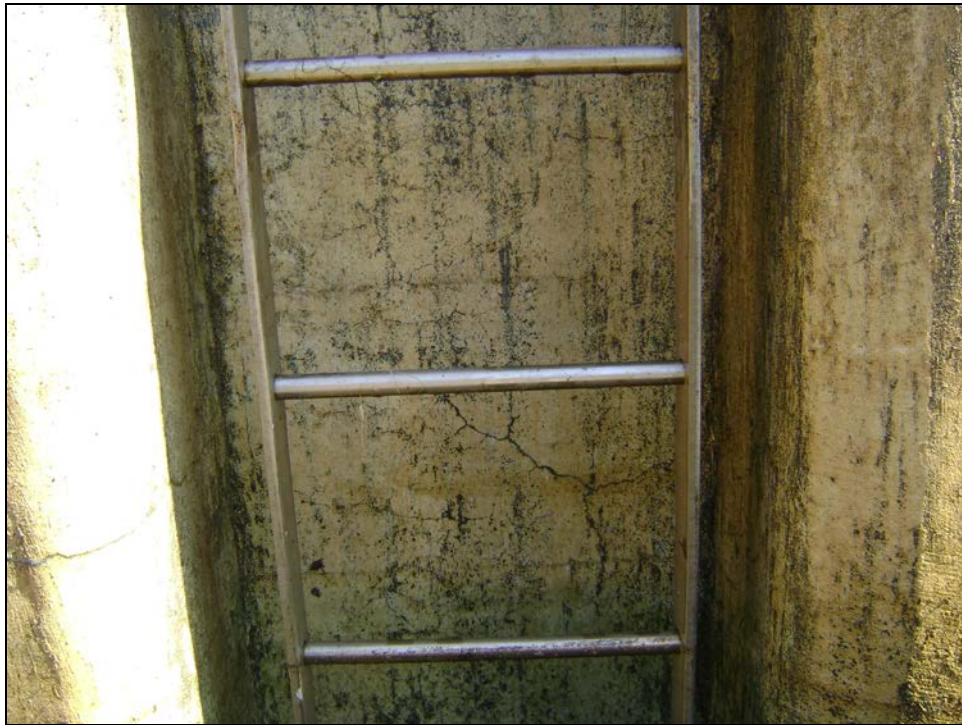
Figure 14. Photograph of the cracked shotcrete surface at S65A. Crack width ranges from hairline to 1/8-inch wide. After South Florida Water Management District, Memorandum on S-65 and S-65A Concrete Repair Cracks, February 14, 2012.
