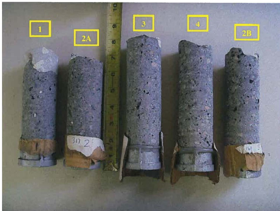
Figure 11. Photograph of the shotcrete cores from S-61 Navigational Lock that indicate voids and separation through the concrete substrate and shotcrete interface. 39
