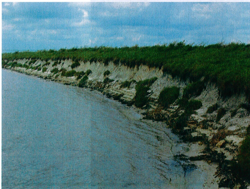
Erosion of internal L-8 Reservoir Embankment
