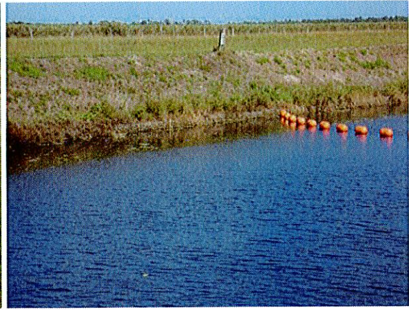
Downstream – South Bank – Gabion
