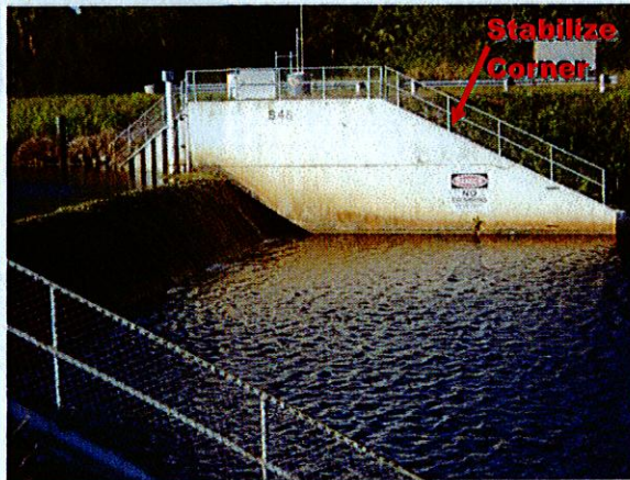
Downstream - N Bank – Stabilize Corner
