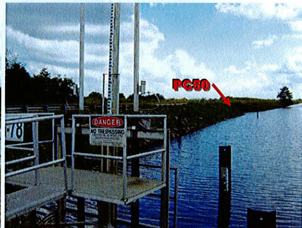
Upstream – E Bank - G78 Structure – PC50 – Stabilize to Existing Riprap
