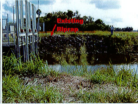
Upstream – S Bank – Existing Riprap
