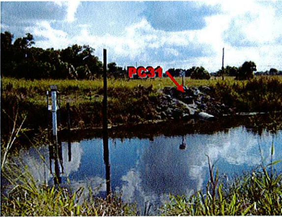
Upstream – Both Sides – Stabilize from End of Existing Riprap to west side of PC31
