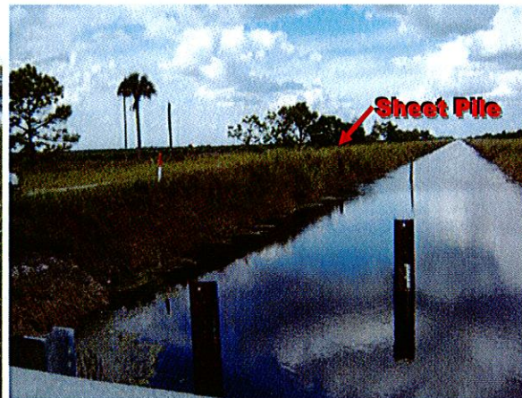
W Bank – Stabilize: Culvert to Sheet Pile
