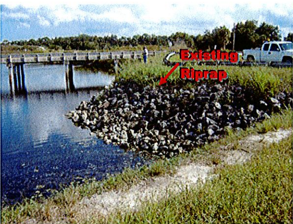
Downstream – S Bank - Existing Riprap – Stabilize from Riprap to Carlton Overpass
