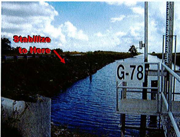
Upstream – E Bank - G78 Structure – PC50 – Stabilize to Existing Riprap
