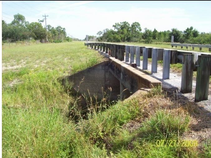
Bridge Structure ID: 214 Watershed: GB Photo # 100_0469
