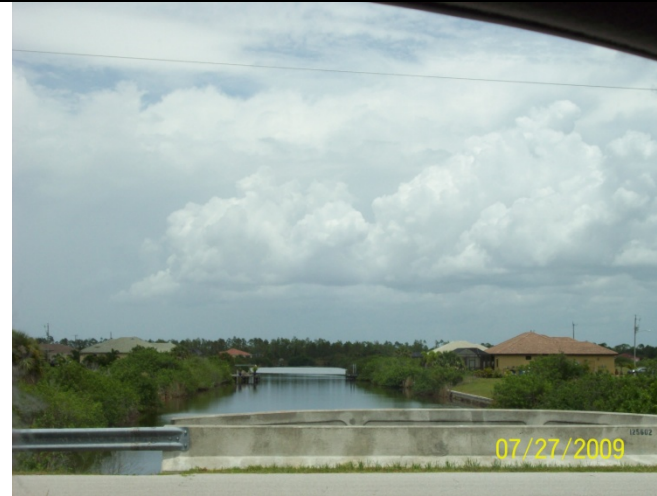
Bridge Structure ID: 229 Watershed: LV Photo # 100_0497
