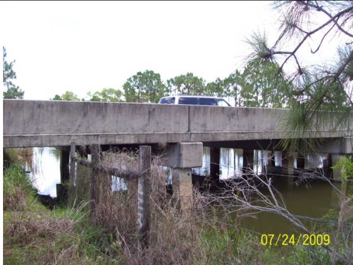
Bridge Structure ID: 142 Watershed: GSE1 Photo # 100_0319
