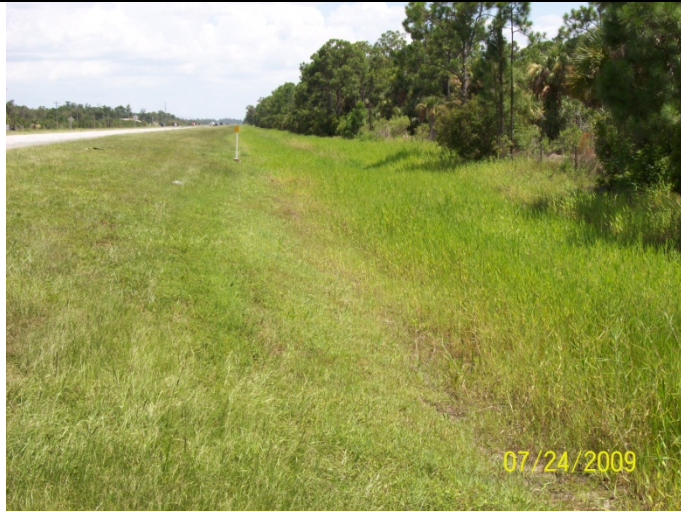
Swale/Ditch Structure ID: 147 Watershed: DC Photo # 100_0334
