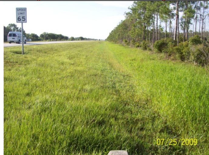
Swale/Ditch Structure ID: 153 Watershed: DC Photo # 100_0357
