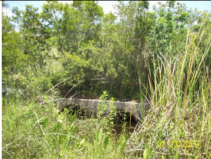
Culvert Structure ID: 113 Watershed: GSE1 Photo # 100_0274
