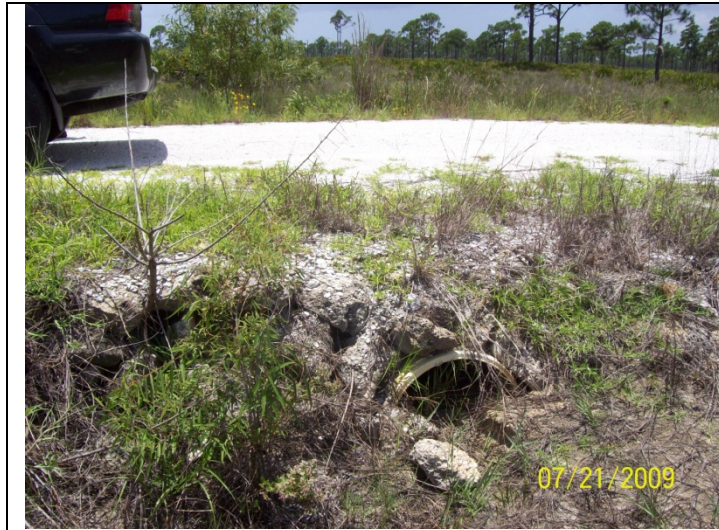
Culvert Structure ID: 36 Watershed: GSE1 Photo # 100_0152
