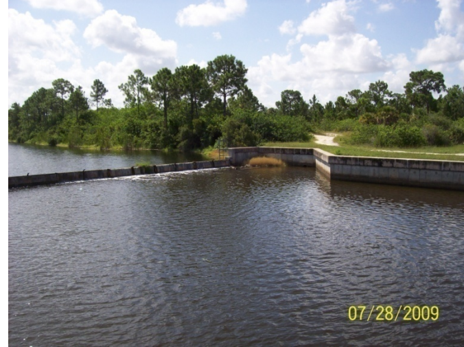
Weir/Drop Structure Structure ID: 253 Watershed: GS Photo # 100_0585
