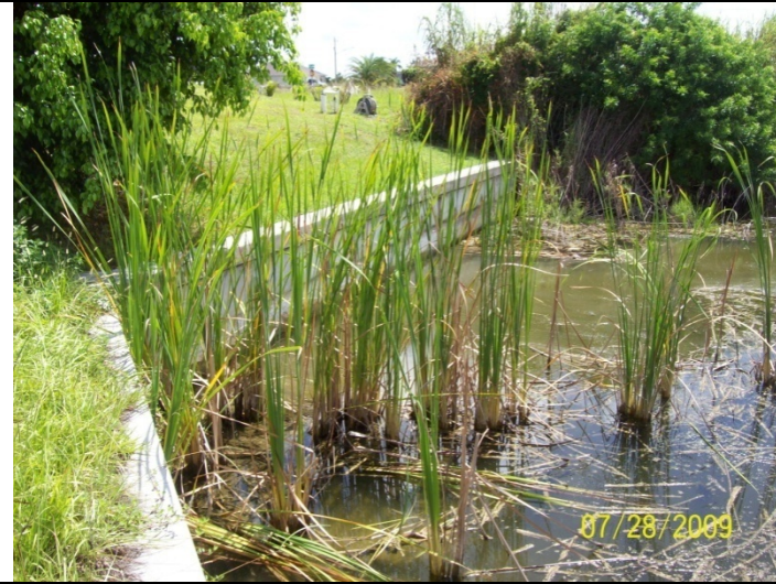
Culvert Structure ID: 253 Watershed: GS Photo # 100_0601
