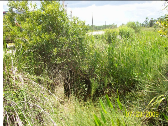
Culvert Structure ID: 120 Watershed: GSE1 Photo # 100_0283
