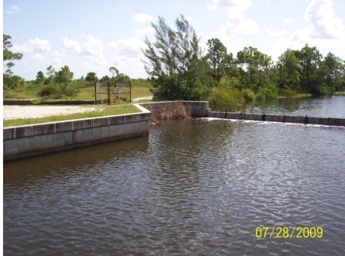
Weir/Drop Structure Structure ID: 253 Watershed: GS Photo # 100_0586
