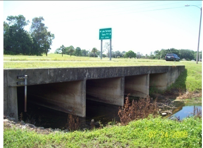
Bridge Structure ID: 148 Watershed: GS Photo # 100_0338
