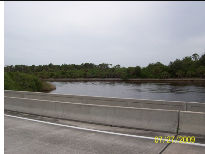
Bridge Structure ID: 231 Watershed: GS Photo # 100_0527
