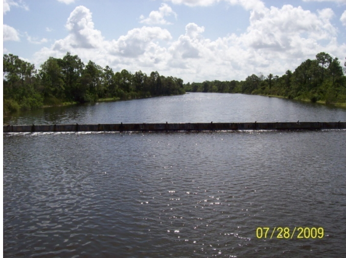
Weir/Drop Structure Structure ID: 253 Watershed: GS Photo # 100_0584
