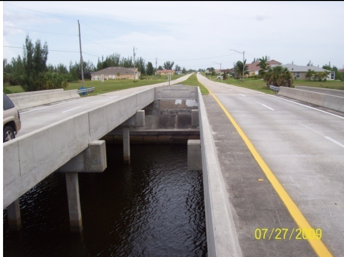
Bridge Structure ID: 231 Watershed: GS Photo # 100_0526
