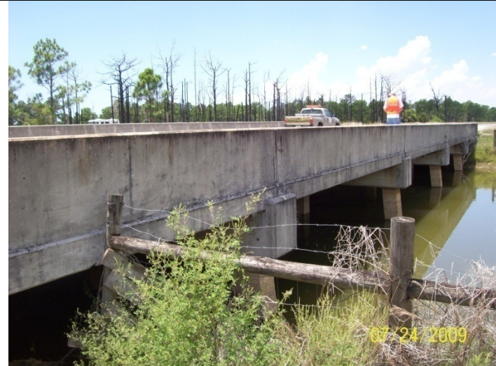
Bridge Structure ID: 146 Watershed: GSE1 Photo # 100_0328
