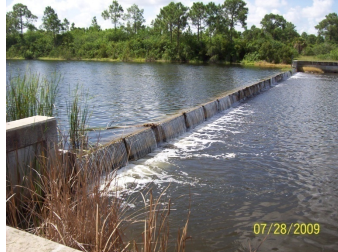
Weir/Drop Structure Structure ID: 253 Watershed: GS Photo # 100_0597
