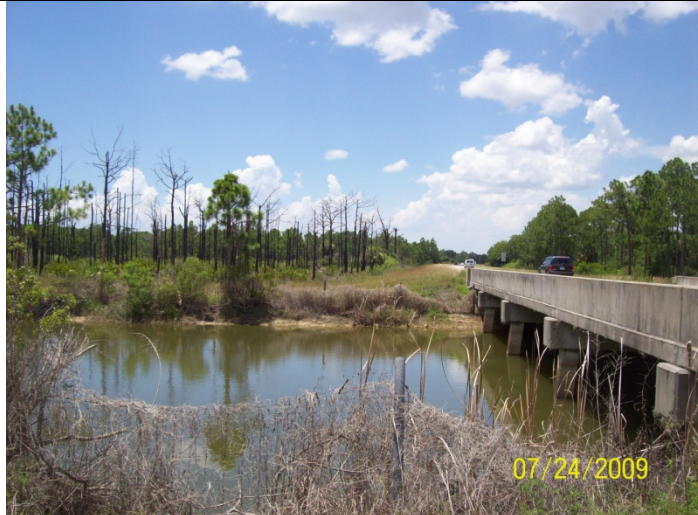
Bridge Structure ID: 146 Watershed: GSE1 Photo # 100_0331
