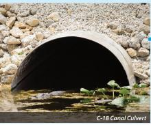
**Culverts:** Structures that allow the flow of water between two areas. They are typically placed under roads or levees.
