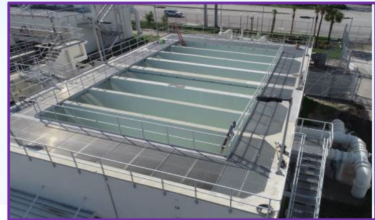
Existing and New Effluent Filters and Chlorine Contact Tanks
