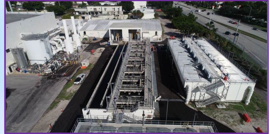
Existing and New Effluent Filters and Chlorine Contact Tanks
