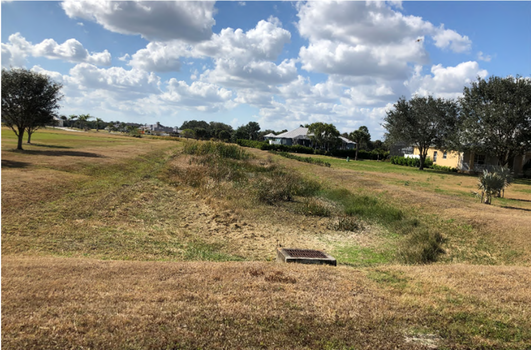
Original Banana Branch Channel (discharge). Looking NW toward the C43 in background. Channel used as residential discharge swale now. Water control structure in photo drains under road and into the new channel of the Banana Branch. – (2/09/21)
