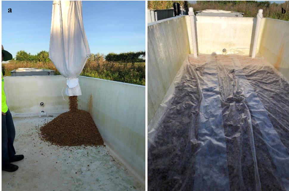
**Figure 3.** a) Red river rock being loaded into mesocosm tank. b) Geofabric covering red rock with 2 PVC sample collection wells at the end of the mesocosm tank.
