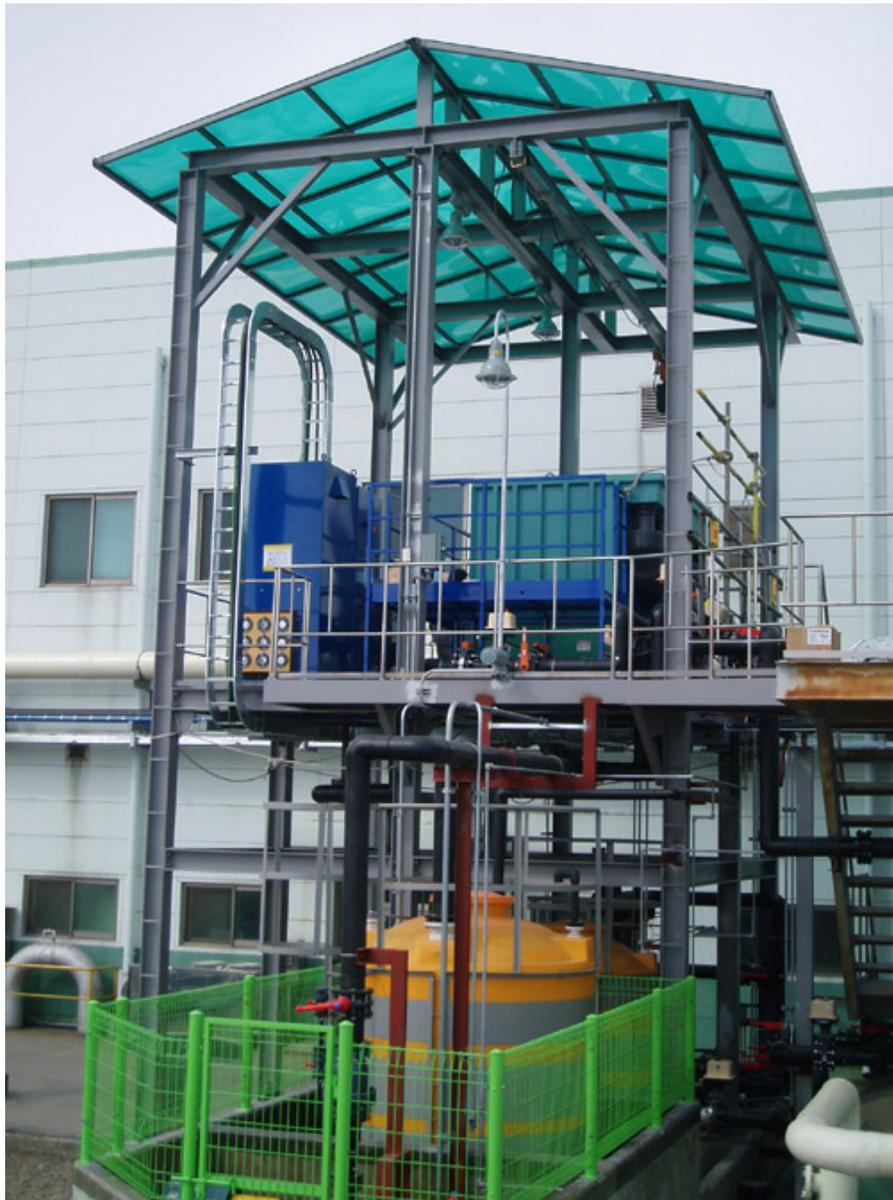
The EC chamber and control panels are blue on the elevated structure. The CIP acid tanks are below.
