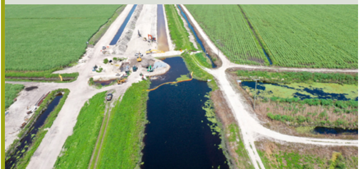
G-341 Conveyance & Related Improvements; Segment #4 Construction. (Photo by SFWMD)
