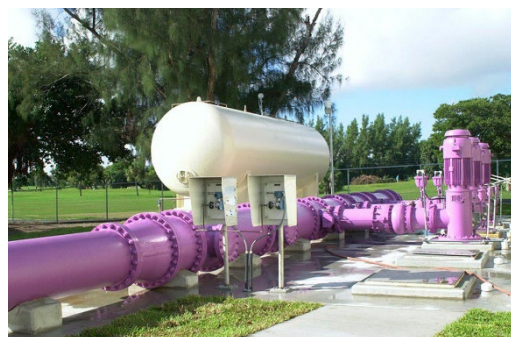
Figure 6-4. Picture of reclaimed water "purple pipes".
