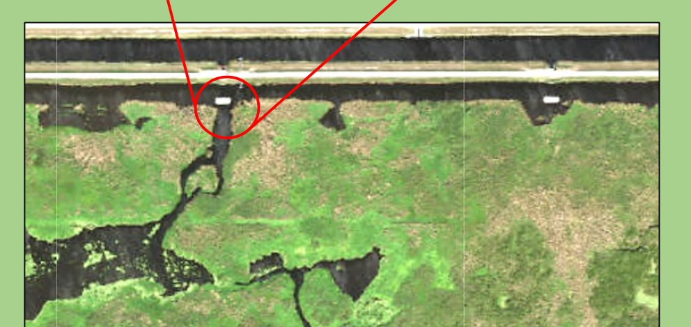
STA-3/4 Energy dissipators located south of inflow structures; inset is a southern view at the G-377B structure
