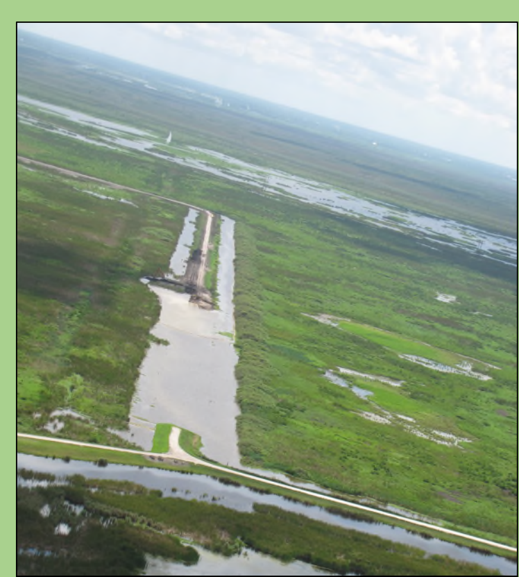
STA-1W East-west Levee removal to reshape Cells 2A and 5B
