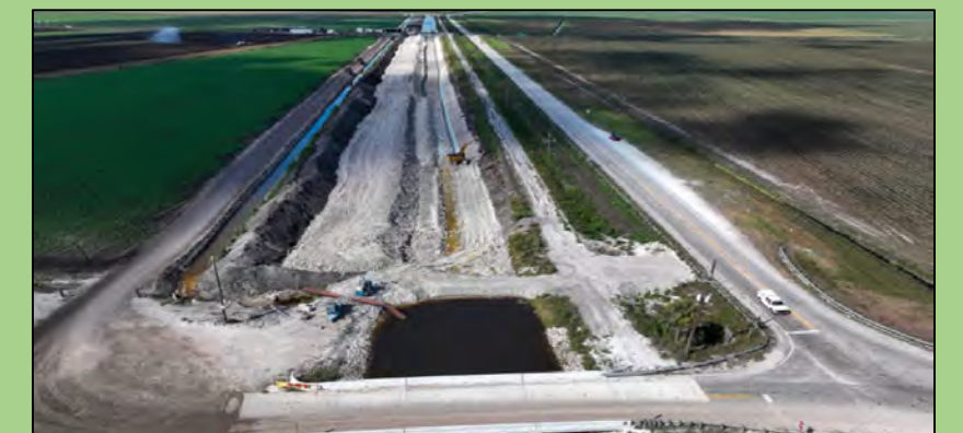
G-341 Related Conveyance Improvements Segment 5 in Bolles East Canal
